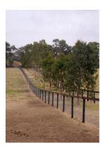
fence made from recycled plastic bottles. Looking very much like timber and expected to last 25-30 years, they are so much cheaper than the iron bark used up until now.
